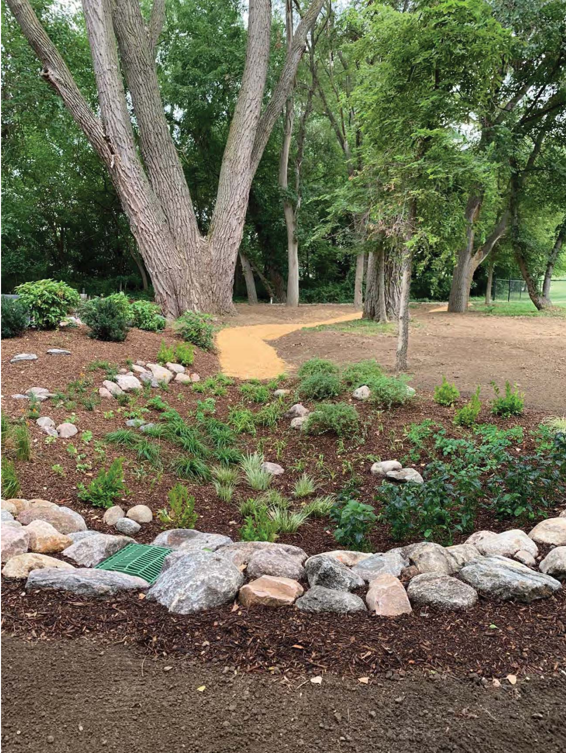
View to the East, with temporary straw matting (for erosion) showing part of proposed dry creek bed #1. Berm to be secured is on the left of the straw in front of the large tree.
