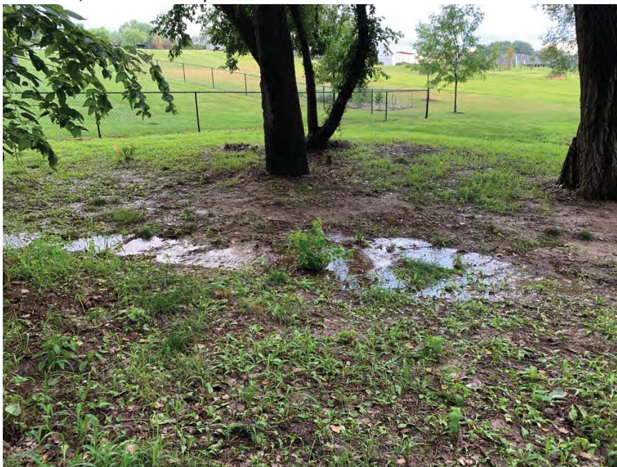
Standing water in area of proposed rain garden (pre-installation).
