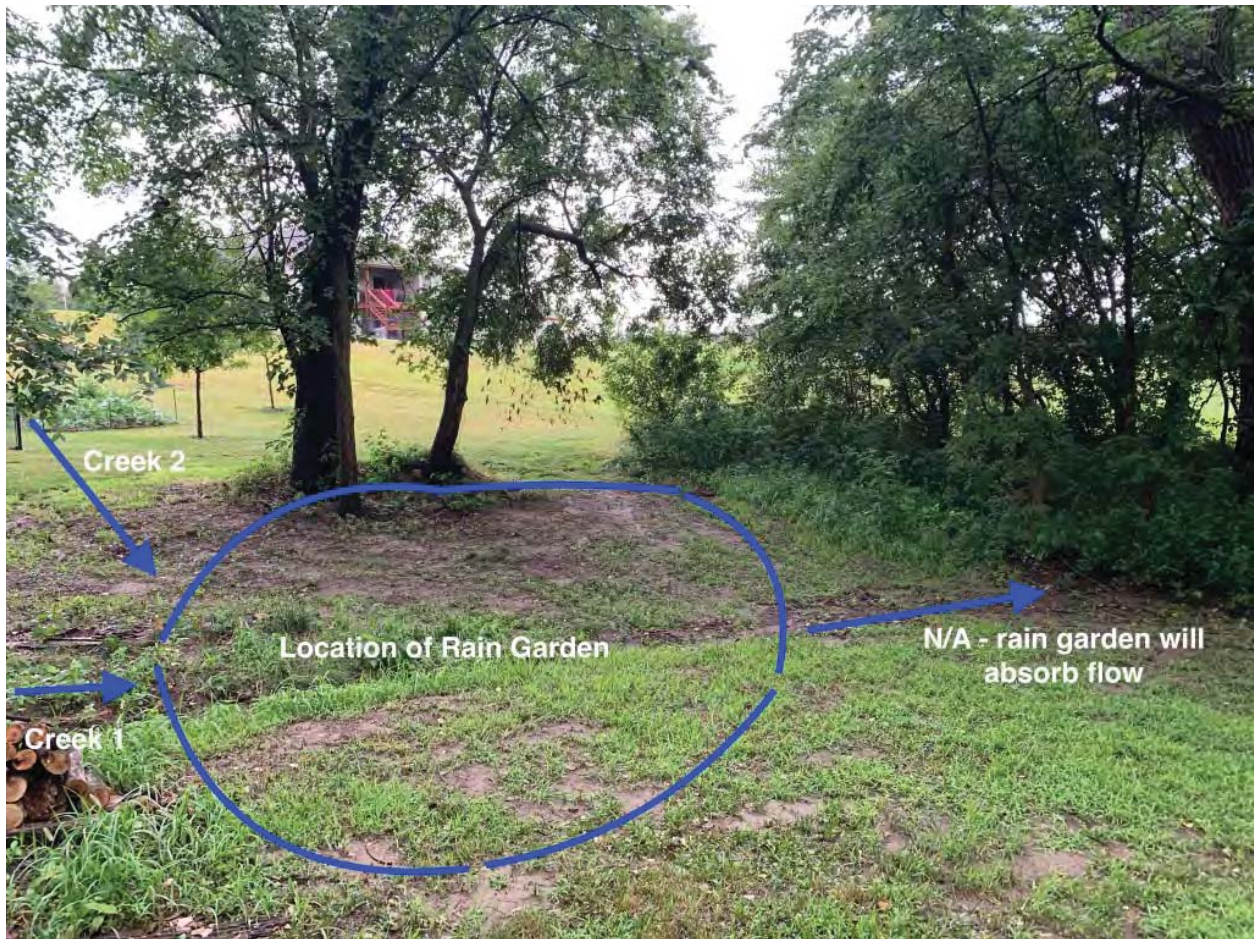
Figure 5: Proposed location of rain garden at the merging of Creek 1 and Creek 2. Update: now installed, see finished pictures above.
