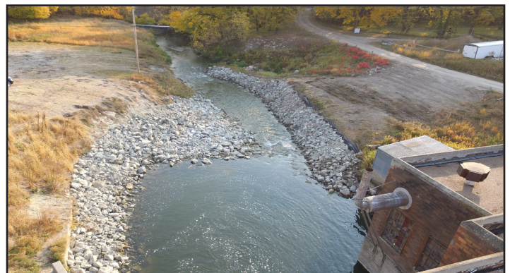
Mill Pond before EWP repairs (top) and after.
