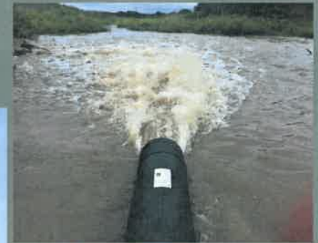
Upper Republican NRD installed the Rock Creek drop structure near Parks to reduce channel erosion due to water releases from the Rock Creek augmentation project.
