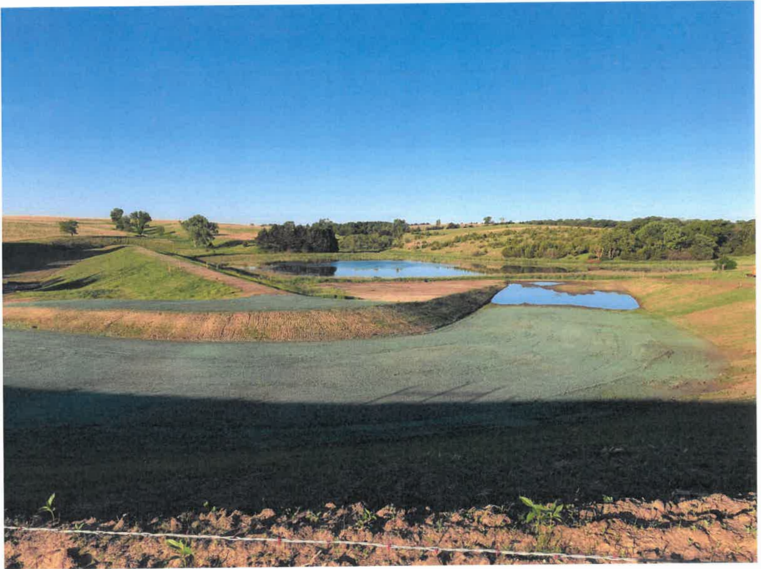
Oak-Middle 82-B – looking south across the auxiliary (emergency) spillway. Note the dam, wetland mitigation area, and that the lake has not completely filled.
