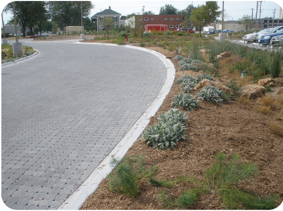
Pervious pavement and bioswale - Antelope Valley
