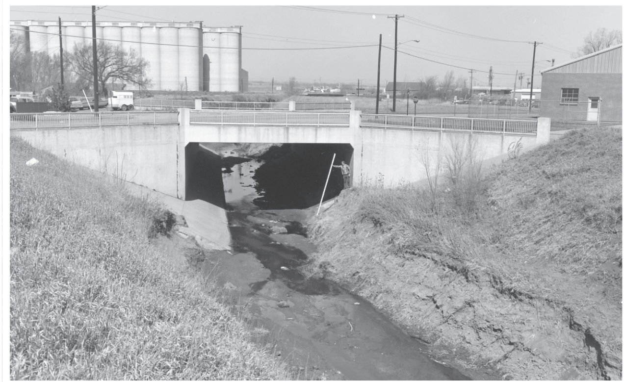
9. Dead Mans Run channel at 33rd and Baldwin bridge looking northwest. March 1967.
