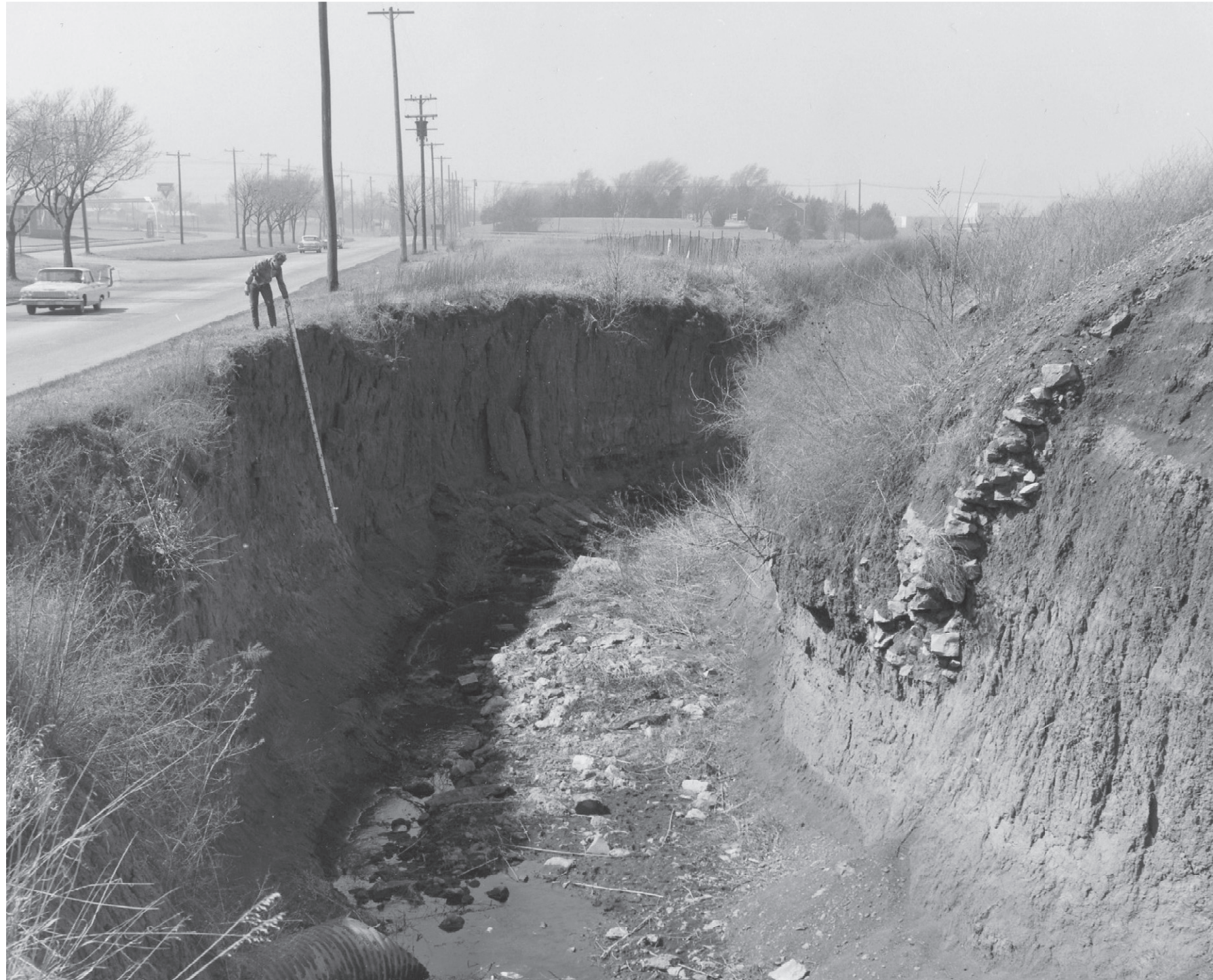
33. Dead Mans Run channel looking west from Missouri Pacific bridge. 0 Street at left. Note proximity of eroded channel to roadway. Storm sewer outlet at left foreground. March 1967.
