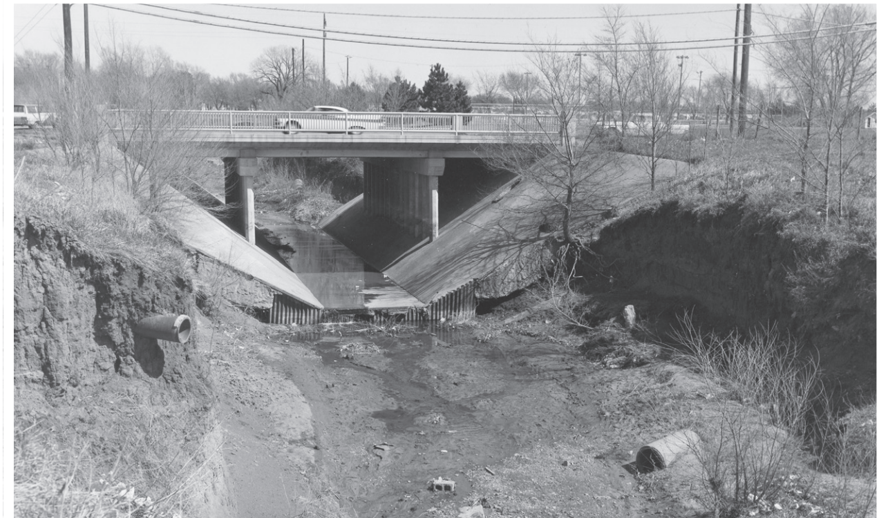
2---Dead Mans Run channel looking east. 48th Street bridge. Note exposed sheet piling cut off wall and cast iron water main at right immediately downstream from cut off wall. Pipe extending from bank at left is drain tile from field. March 1967.
