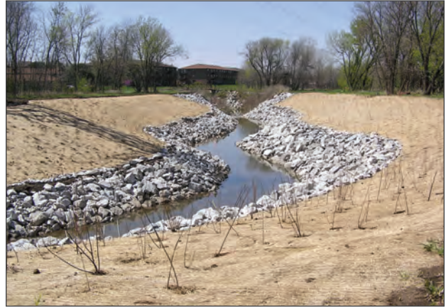
Urban stream improvement
