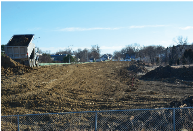
The dry and warm fall of 2017 extended the NRD's construction season (see page 6).
