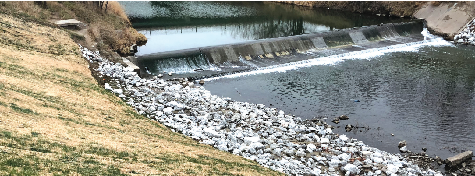
This newly-repaired weir on Oak Creek, near First Street, in Lincoln, decreases the slope of the waterway to help avoid erosion.
