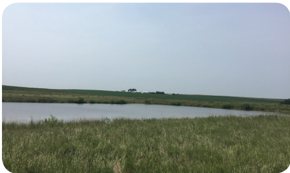
After: Finished Dam
