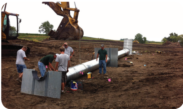
During: Building Dam
