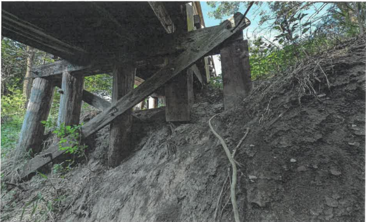
Bent 4 pile 3 and 4 rejected, 1 and 2 previously posted
