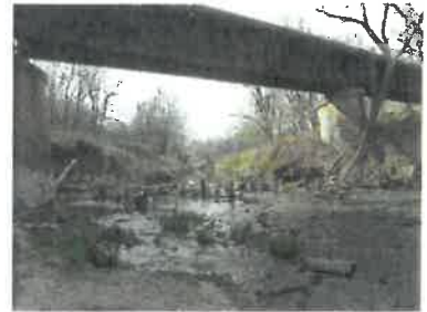
Figure 7-16: Knickpoint Downstream of old Railroad Bridge Knickpoint
